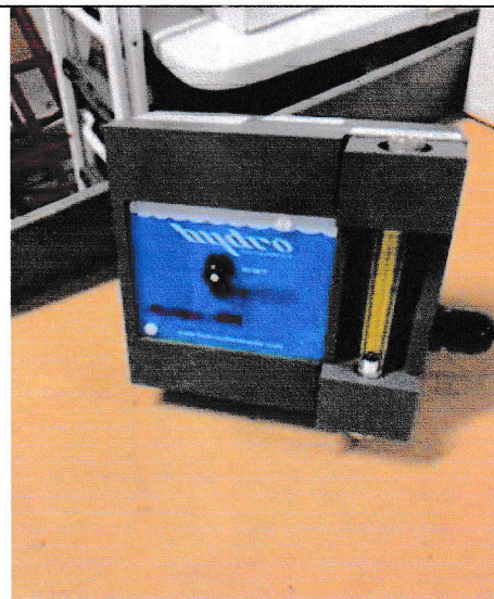
Model VRH-100-CL2-MS Vacuum Regulator
