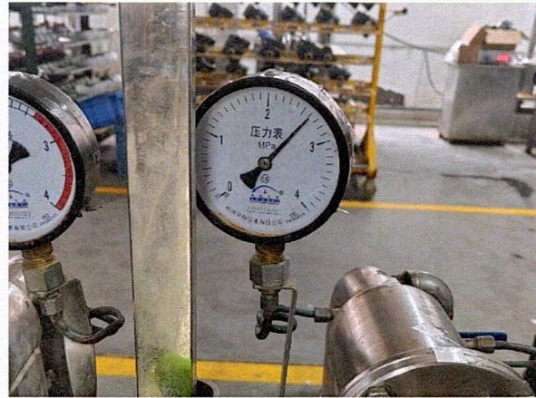
Fig 19. Static hydraulic pressure test
